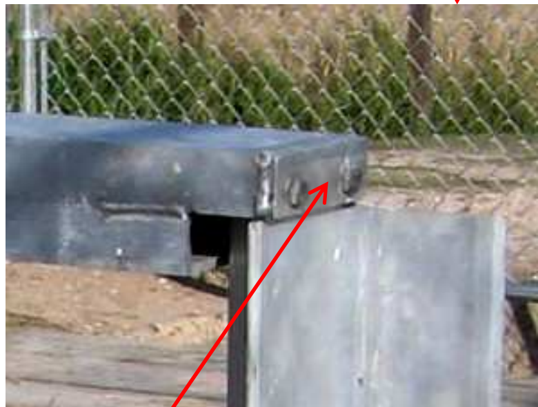
6 inch x 2 inch aluminum end plate
