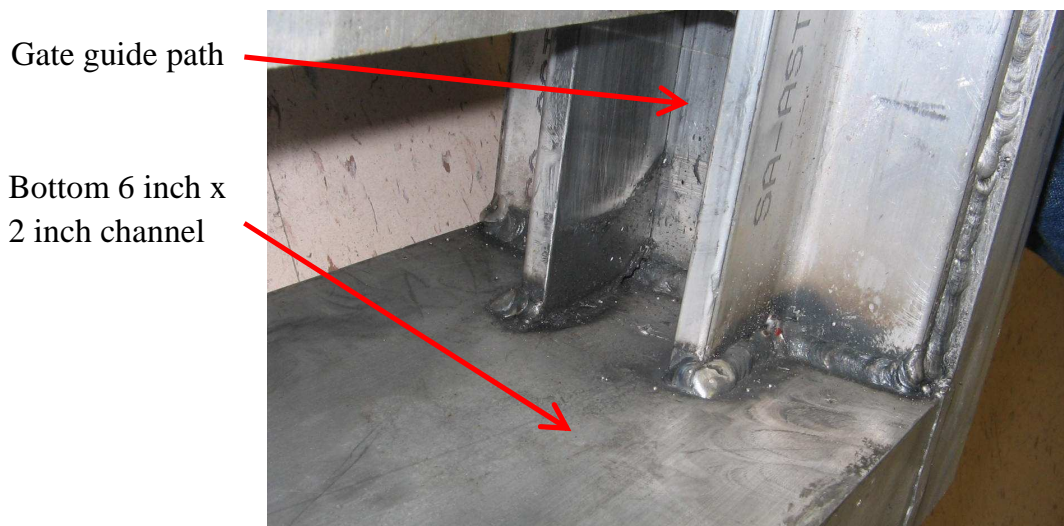
Figure 8. Construction of bottom of gate frame.
