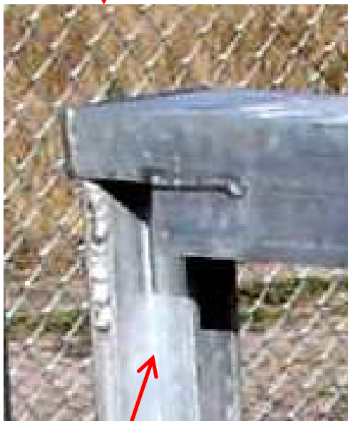
2 inch x 2 inch aluminum angle
